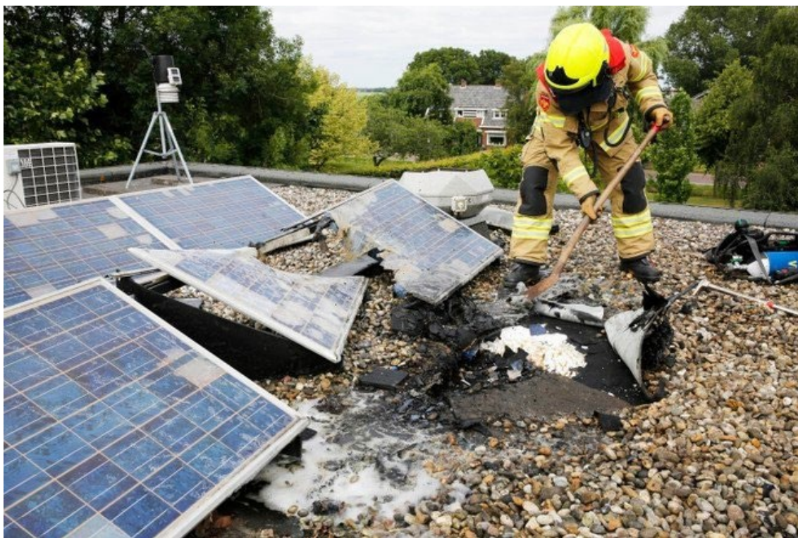
Figure 7 Fire on roof of Opmeer town hall (source: www.noordhollandsdagblad.nl )
