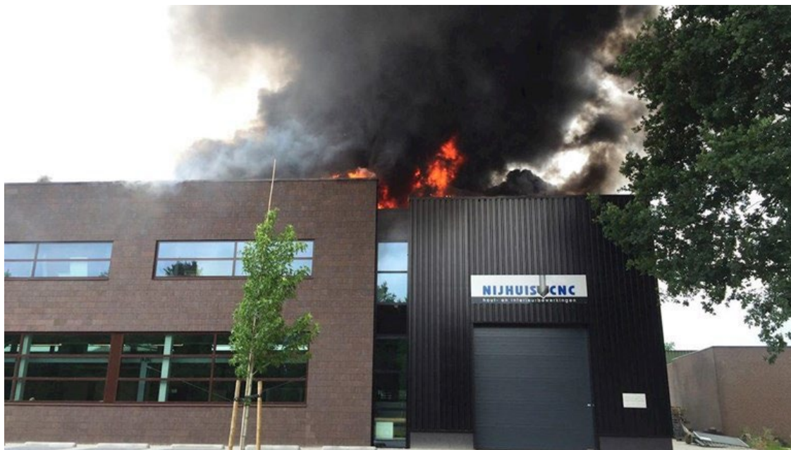
Figure 1 Fire on the roof (source: www.rtvooost.nl )
